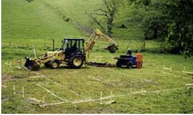
Marking out and starting foundations
