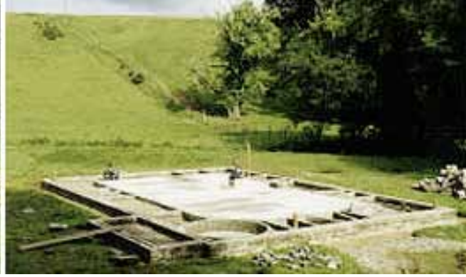
Marking out and starting foundations
